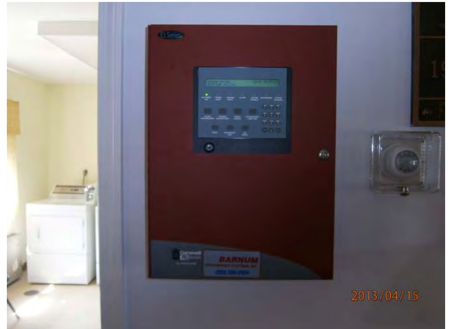
18. Fire system control panel
